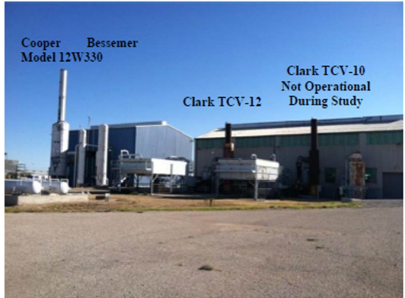
Figure 2-6. Station 102 Compressor Buildings and Stacks
