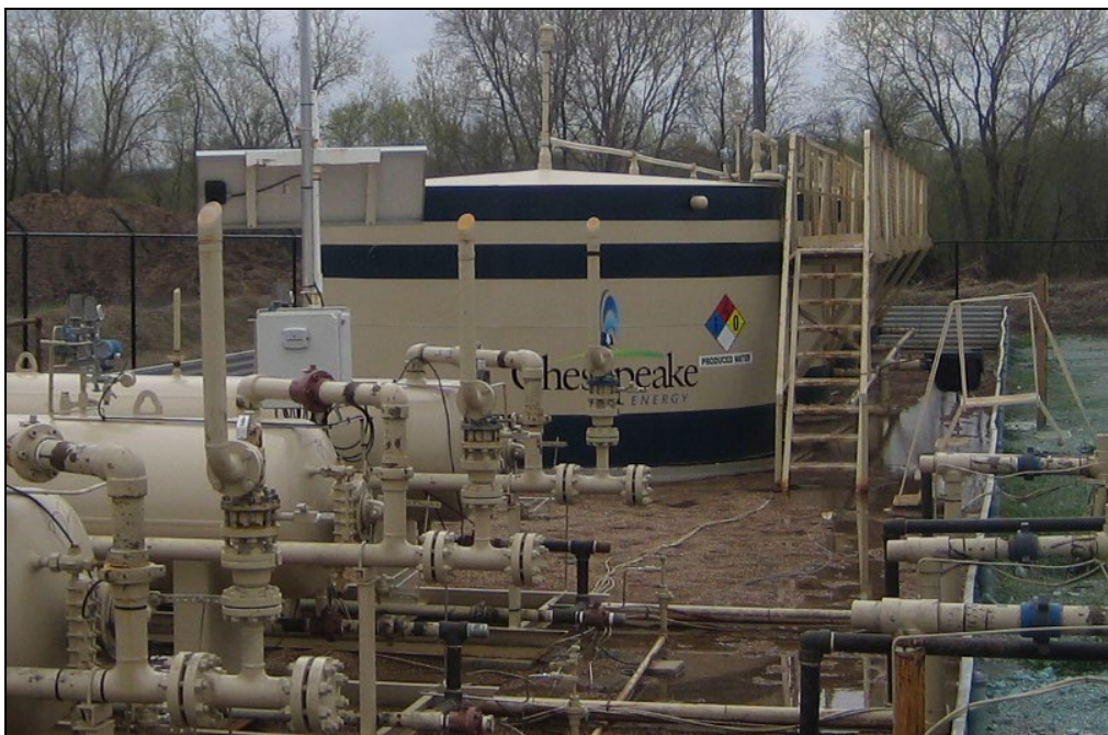
Figure 3-15. Produced Water Tanks
