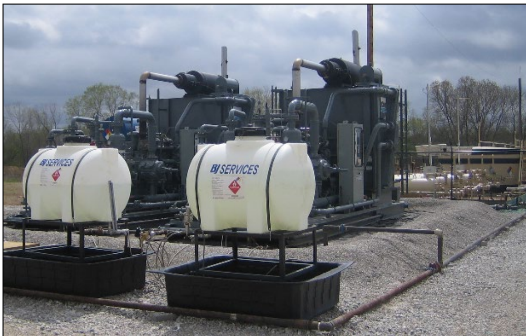
Figure 3-17. Wellhead Compressor Engines
