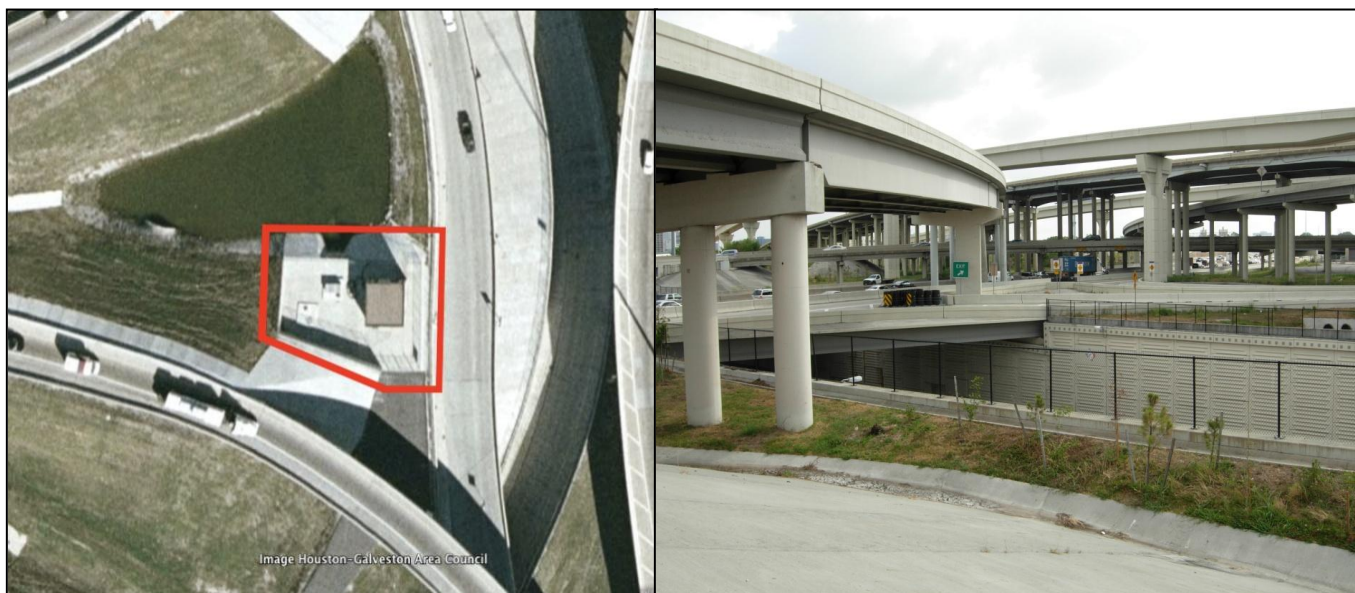
Figure 4. Left: Enlargement of measurements location. Right: Partial view of the Highway junction.
