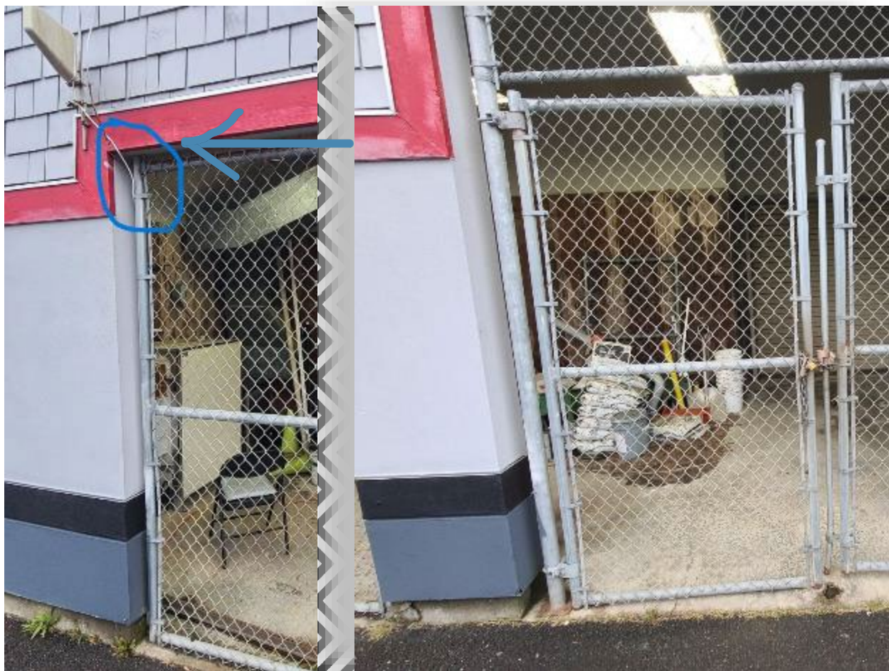
Figure 6: Exterior view of the enclosure which houses Quinault's Nephelometer. The area where Quinault's Radiant Research M903 nephelometer's air intake is located is circled. The installation of the collocation-dedicated Nodes here would likely be easiest to complete by fastening the Nodes to the top of the chain link fence, on the interior side of the fence, in a row adjacent to the Nephelometer's air intake, spaced by a foot or so each. NOTE: roughly 10 feet of horizontal space not pictured lies between the two photos stitched together for this figure.
