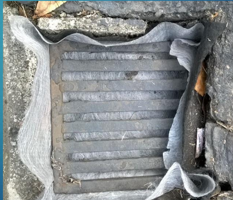
2 layers of Filter Fabric under storm grate
