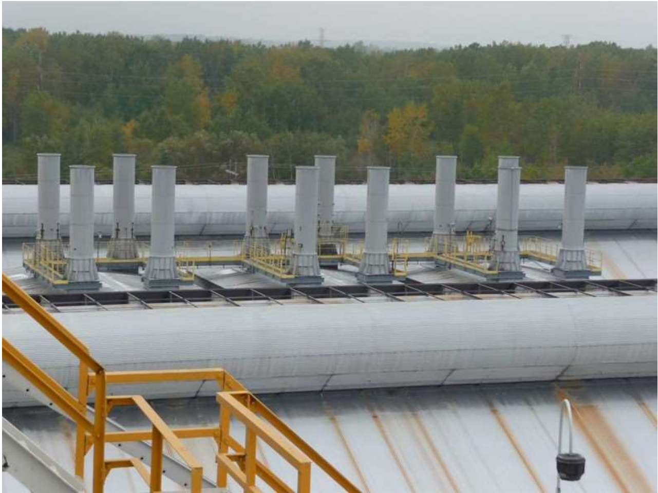
Figure 3-4: Photo of one of the three potline dry scrubber stack clusters at Massena Operations
