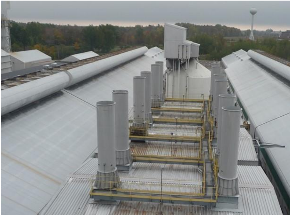
Figure 3-1: One of the Three Potline Dry Scrubber Stack Clusters - Heat Generated by the Potlines
