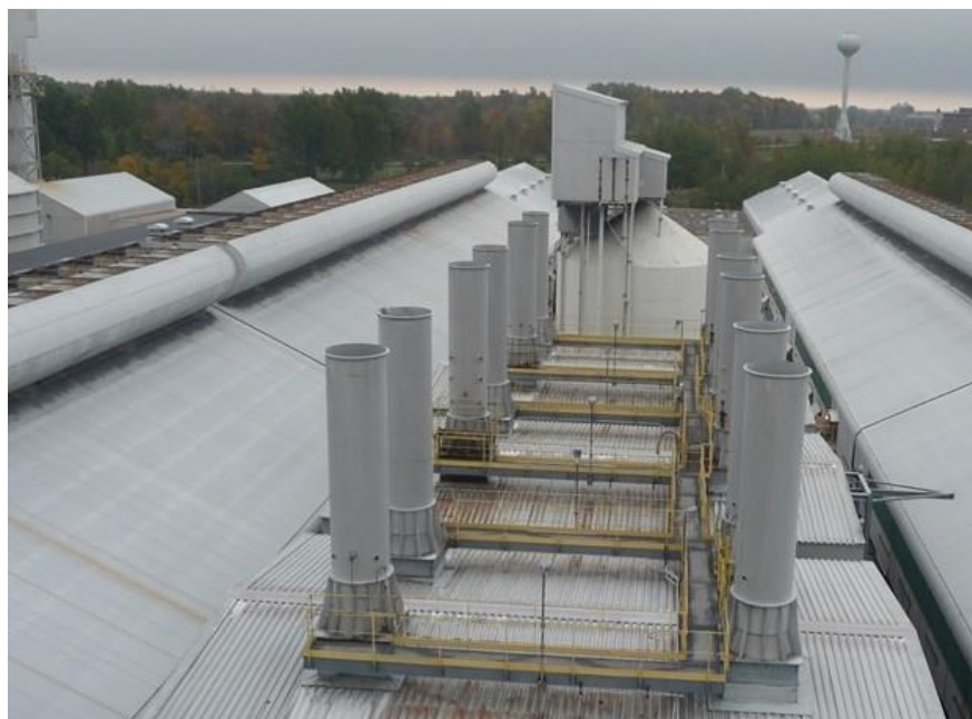
Figure B-1: One of the Three Potline Dry Scrubber Stack Clusters - Heat Generated by the Potlines
