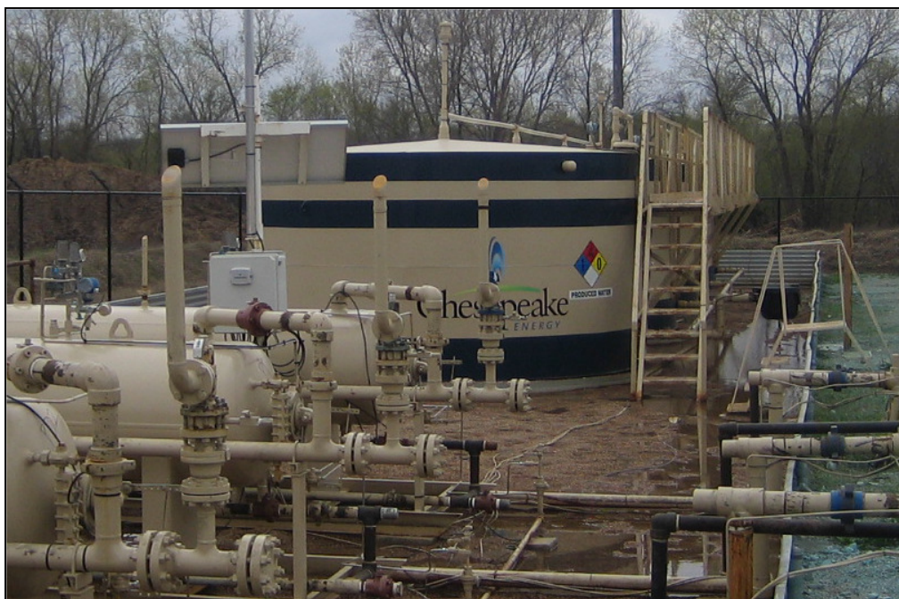
Figure 3-15. Produced Water Tanks
