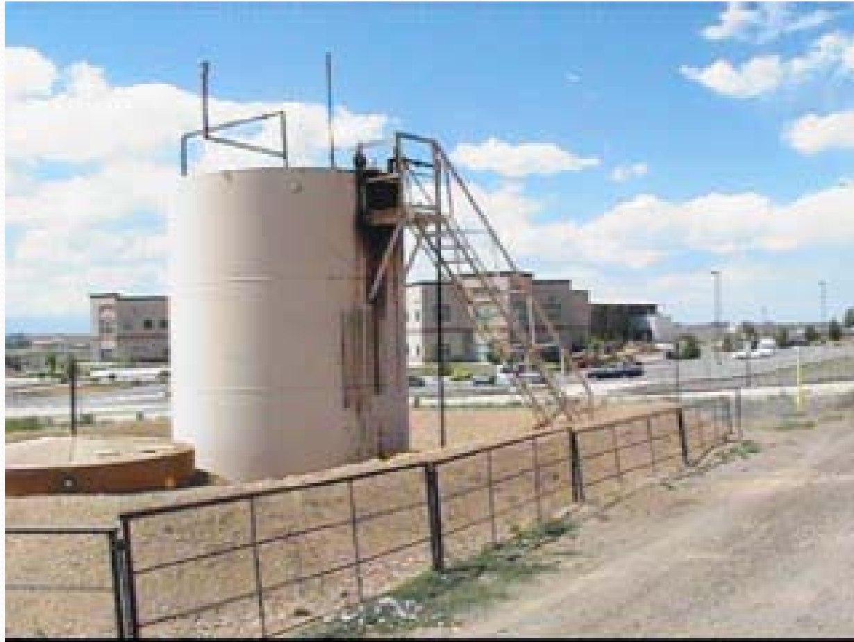
Production Well Pad Condensate Tank next to a Bible School
