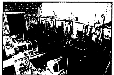
A wastewater treatment plant in Oxnard, California, U.S.A., operates on sewage digester gas. These Waukesha P9390 engine generator sets provide plant power and utilize waste heat to heat digesters. The engines were fitted with the PSC system and are achieving less than 50 ppmv at 15% \text{O}_2 , \text{NO}_x levels. The systems operate in Ventura County, California, U.S.A., which has some of the most stringent emission requirements for internal combustion engines in the U.S.
