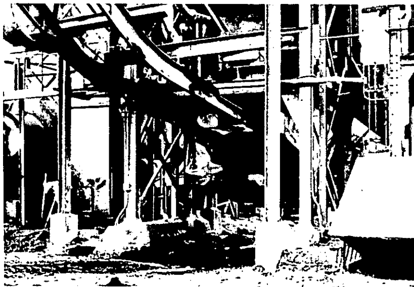
SKIP HOIST IN RECEIVING POSITION UNDER SHROUD
