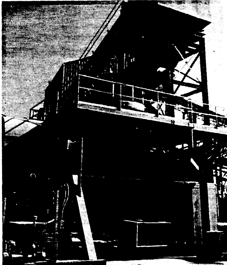
Figure 4. Side View of 7' Crusher
