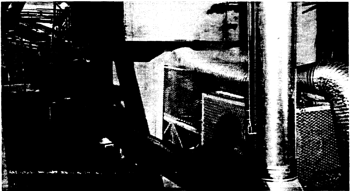
Figure 8. Crusher Outlet Enclosure
