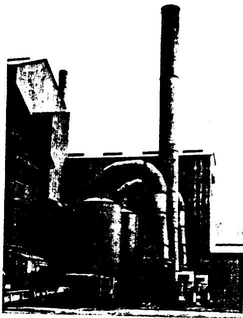
Fig. 3—High energy wet scrubber installation on 25-mw FeCrSi furnace.
