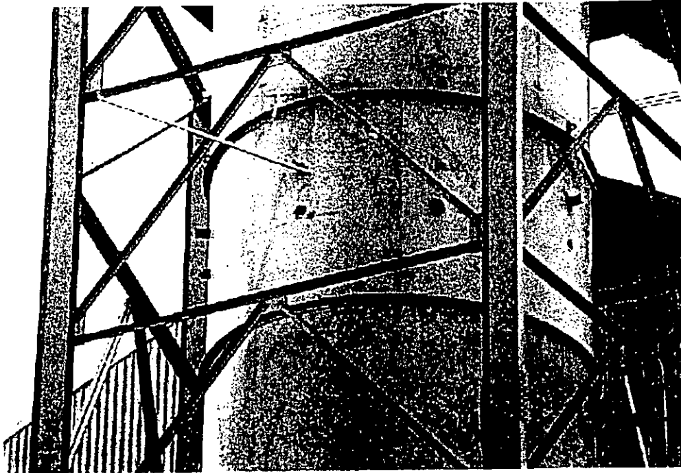
Figure 2. Melt Shop - Before Slag Quenching - Baghouse Inlet Sampling Location
