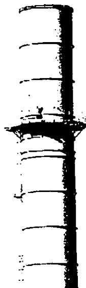
Figure 5. Melt Shop - EAF - Stack Sampling Location
