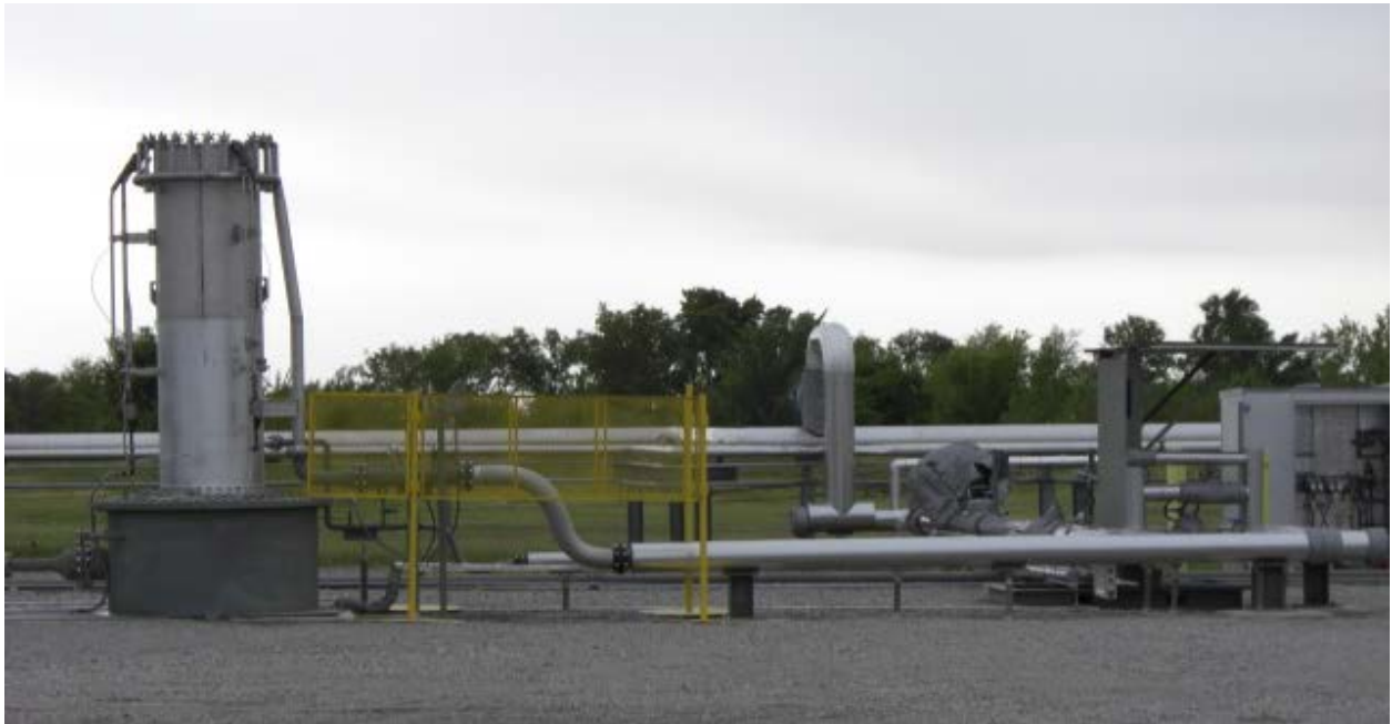
Figure B-4. Steam lines for the steam-assisted flare burner.
