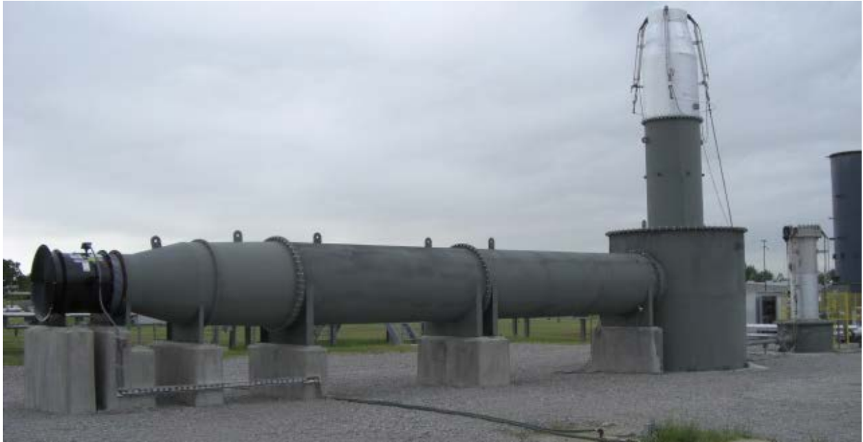
Figure B-7. Air supply for air-assisted flare burner
