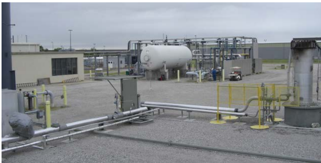
Figure B-9. Control room (with glass windows) and vent gas supply system (center background)
