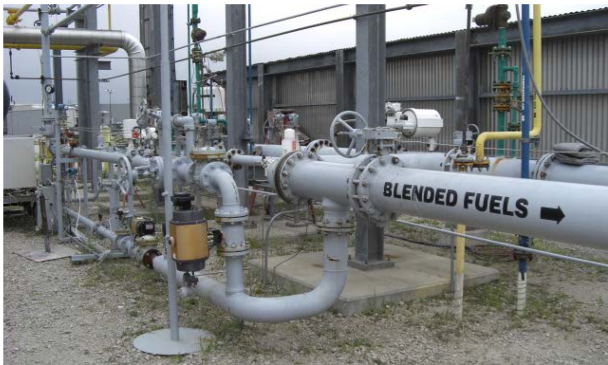
Figure B-10. Piping for flow control, mixing and measurement of the vent gas supply
