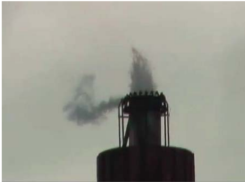
Figure 3.3-1: Steam Leak at Shaping Steam Ring
