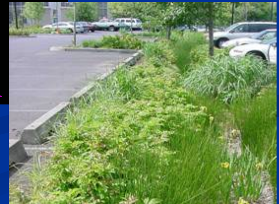
Parking Lot Swales
